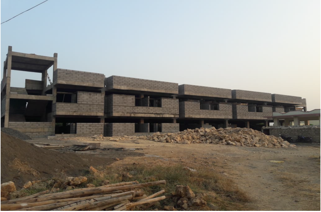
LADIES HOSTEL—UNDER CONSTRUCTION
