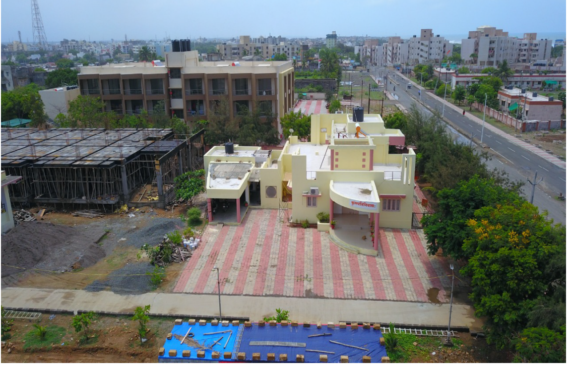
VICE-CHANCELLOR'S BUNGLOW & GUEST HOUSE UNDER CONSTRUCTION
